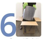
Remove old filter & old prefilter from unit & place into empty box
